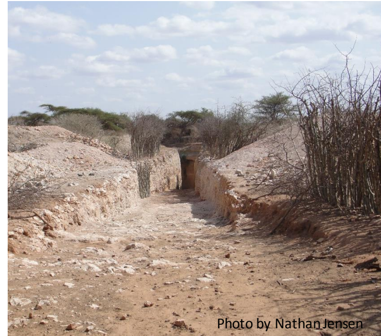
Excavation leading down to an ela (well) in the Borana region.
